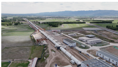
图 13 超高速低真空管道磁浮铁路全尺寸试验平台 Fig. 13 Full-scale test platform for ultra-high-speed low-vacuum tube maglev railway
